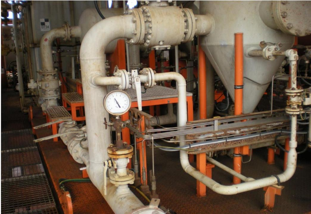
**Plate 1:** Hydro-cyclone De-sander and De-oiler Unit
